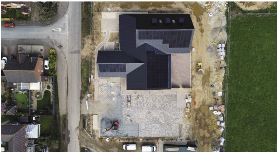
Aerial view of the work progressing on the community centre
